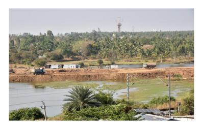
Bhimenahalli Lake, near Bidadi, has been divided into two by a 150-metre-wide earthen dam, upon which foundations for pillars are being laid. DH
